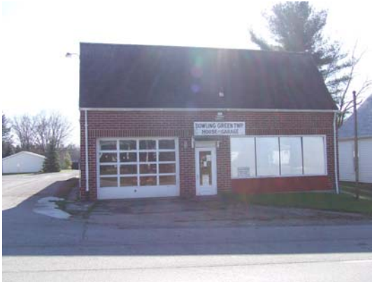
Bowling Green Township House and Garage
